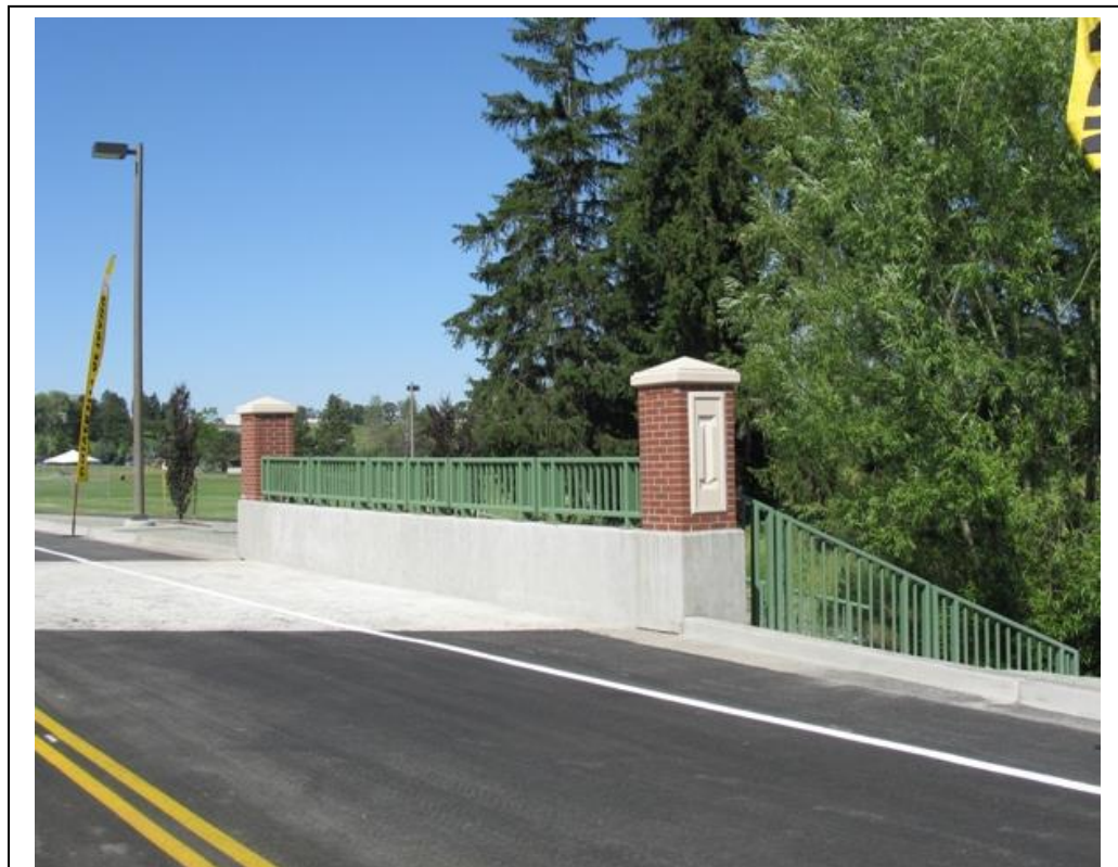
Stadium Drive Cast-in-Place Deck Bridge over Paradise Creek by DPW w/Brick Masonry Pilasters, 2010
