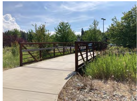
Existing Prefabricated Pedestrian Bridges spanning Paradise Creek.
