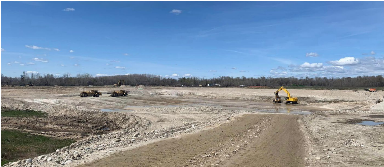
New campground under construction at Eagle Island State Park
