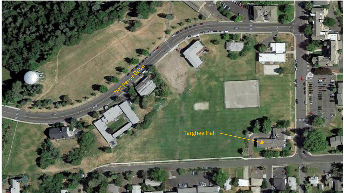
Existing conditions, Nez Perce neighborhood.
