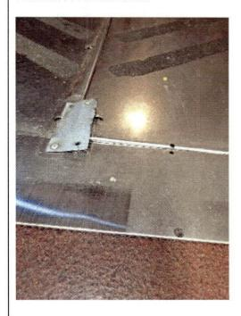
3. The walk-in cooler floor has worn out creating a tripping hazard for staff and causing potential spillage as carts are moved in and out of the area. We have tried to fasten the floor panels down and have been unsuccessful. We have riveted plates over the affected areas, but as seen in the picture above the constant travel over them is causing movement that wearing the fasteners out.
