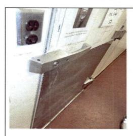
Both unit doors are lockable without exit hardware available on the door interior. This presents entrapment issues that could result in harm to staff if they were trapped inside.
